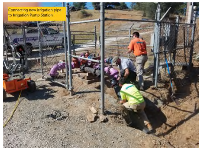
Photo 7 - Modifications to pump discharge piping.
