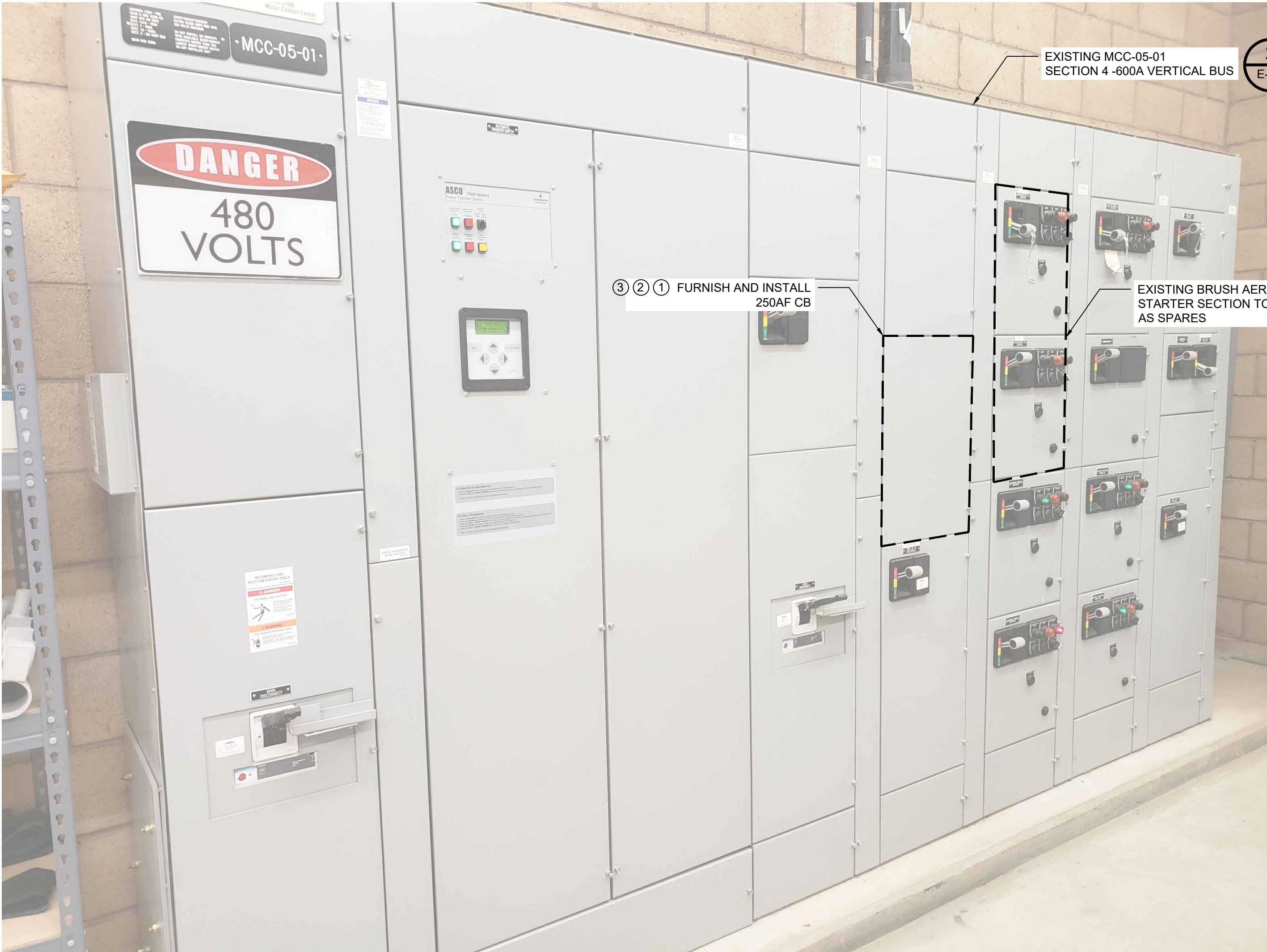
DETAIL 1 EXISTING MCC-05-01 ELEVATION MODIFICATIONS SCALE: NONE
