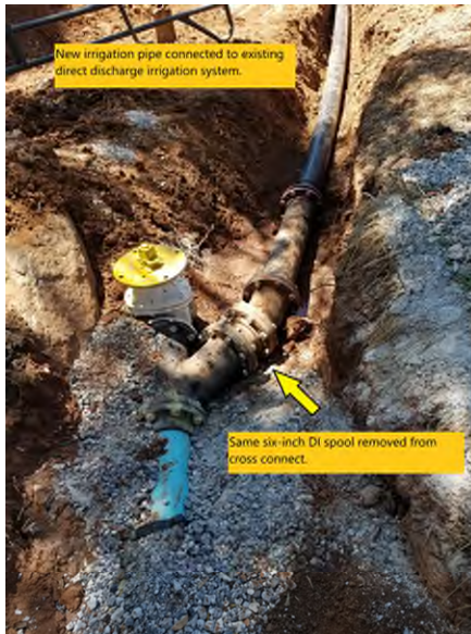
Photo 4 – New irrigation pipe.
