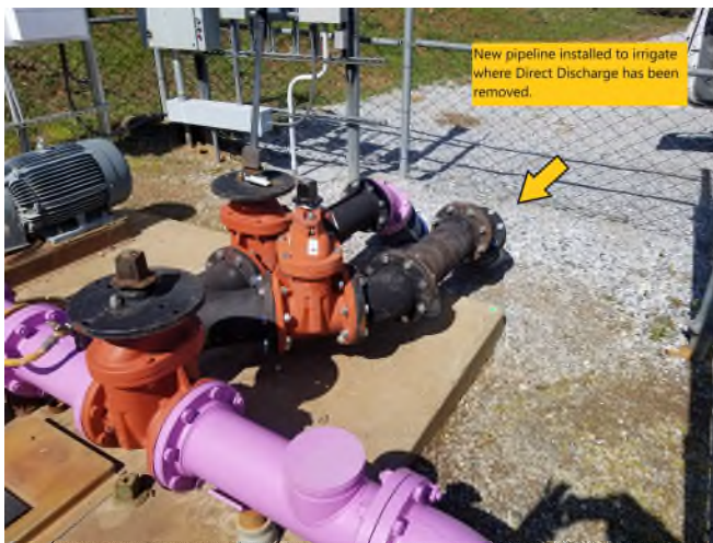
Photo 6 - Modifications to pump discharge piping.
