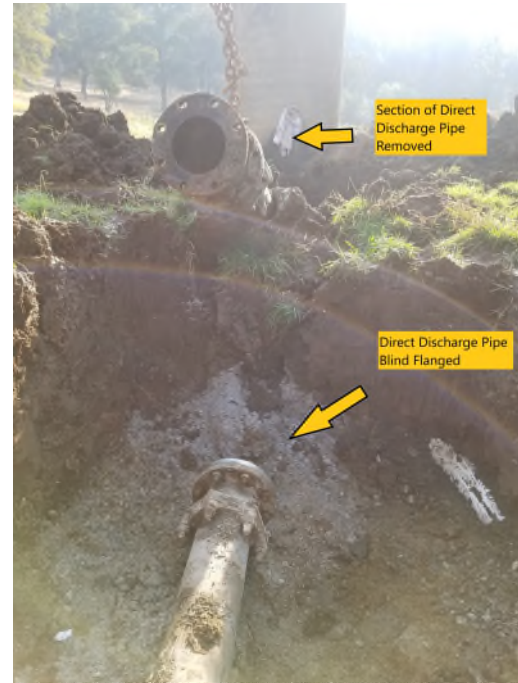
Photo 2 – Section of direct discharge pipe removed and direct discharge pipe blind flanged.
