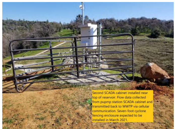
Photo 12 - New SCADA cabinet on top of Reservoir.
