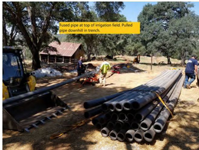
Photo 5 - New irrigation pipe.
