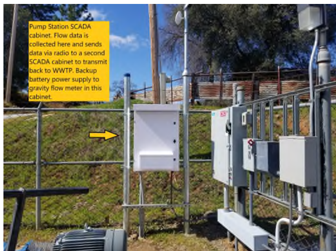
Photo 11 - New SCADA Cabinet.
