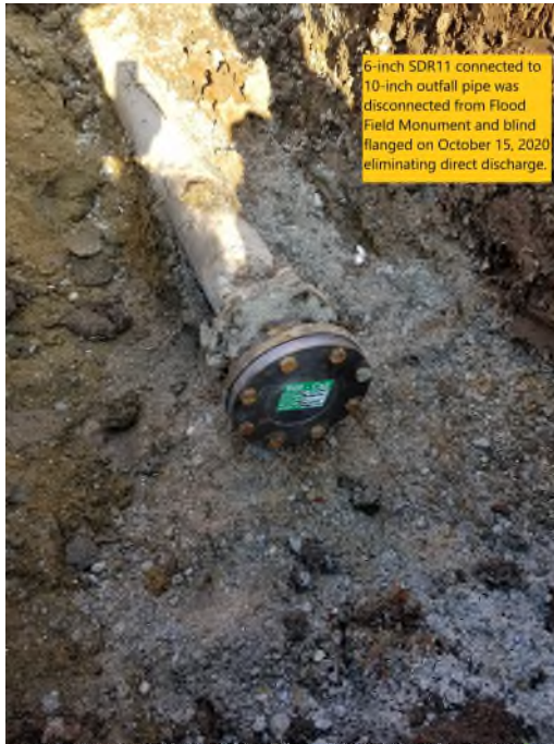
Photo 1- 6" pipe blind flanged and isolated flood filed monument.
